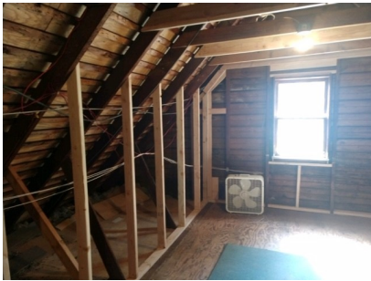
Before the work began
